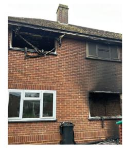
Fire damage to the outside of council house caused by e-scooter battery
